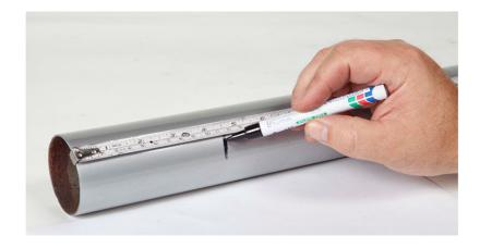
Check the base of the column and mark it to be flush with the fire wall.
