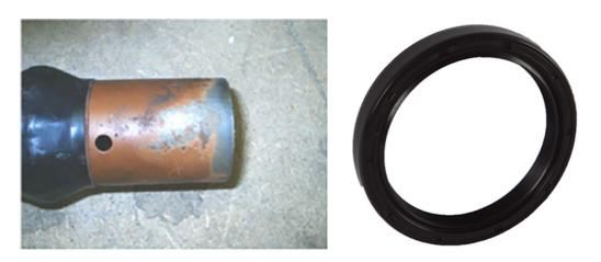
Cut column end off and de burr. Install RRS support ring for inner tube location.
